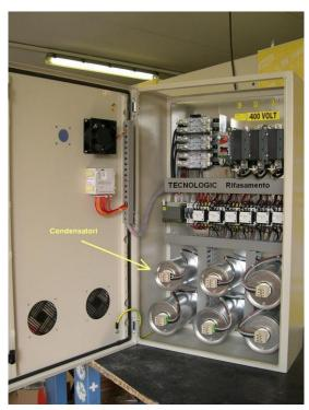
Figure 121: capacitors installed in the electrical panel
